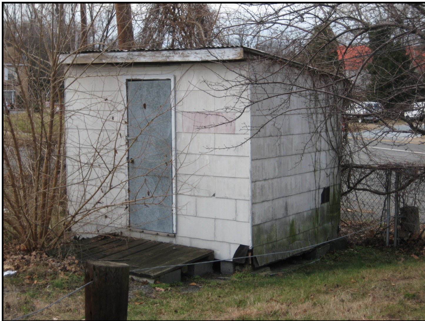
Photo: Shed, Forestville, looking west. (February 2009)
